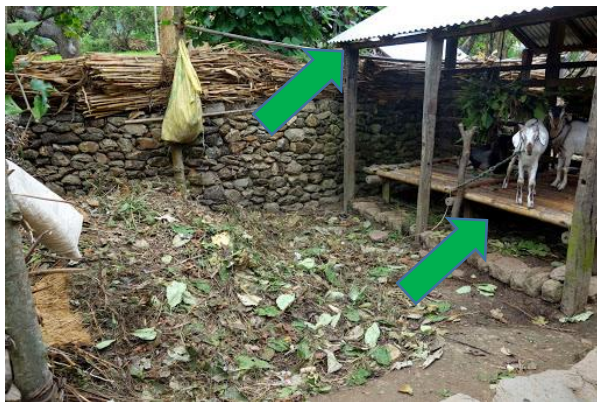
Figure 9: Goat shack with elevated floor and tin roof. Retrieved from http://www.ewbchallenge.org
